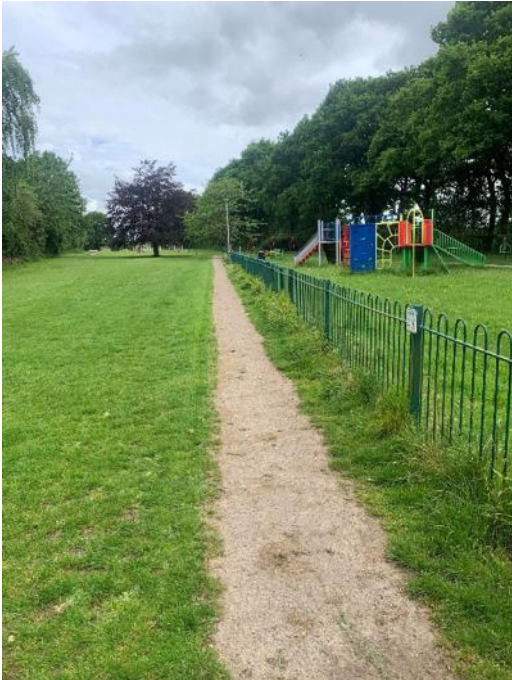
Photograph 9: Footway at Recreation Ground
