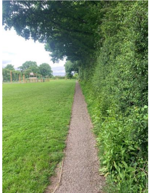
Photograph 10: Footway at Recreation Ground
